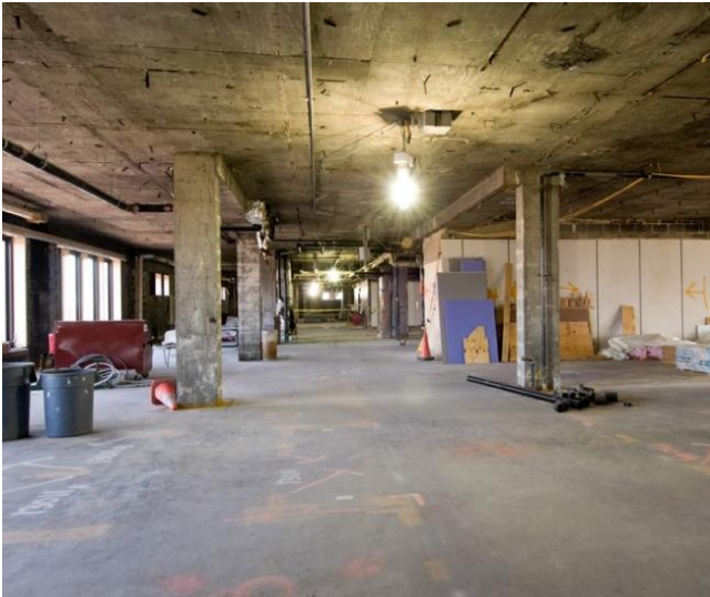
Figure 3: Existing 13 th Floor Demolition
