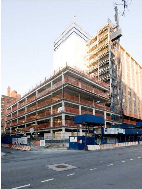
Figure 5: New Building Structural Steel System
