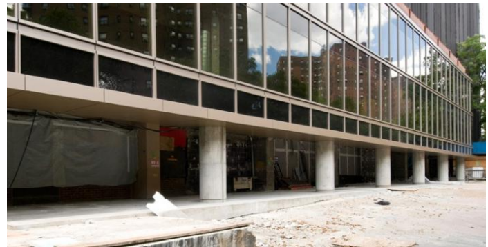
Figure 7: Exterior Support Columns
