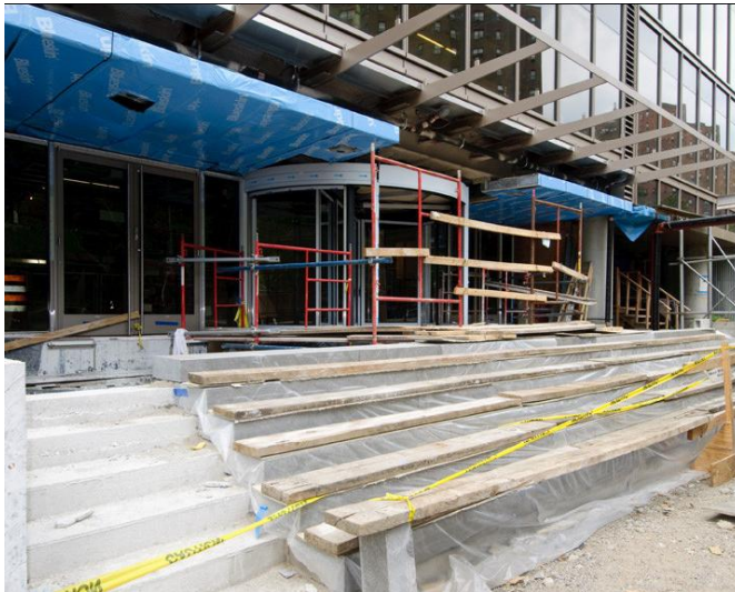
Figure 10: New Main Entrance Granite Stairs
