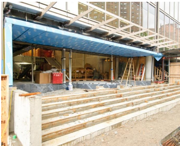
Figure 8: New Main Entrance Stair Base
