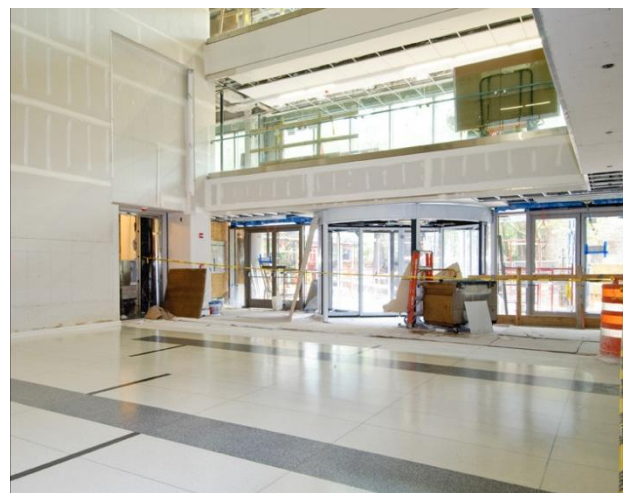
Figure 9: New Atrium Lobby Terrazzo
