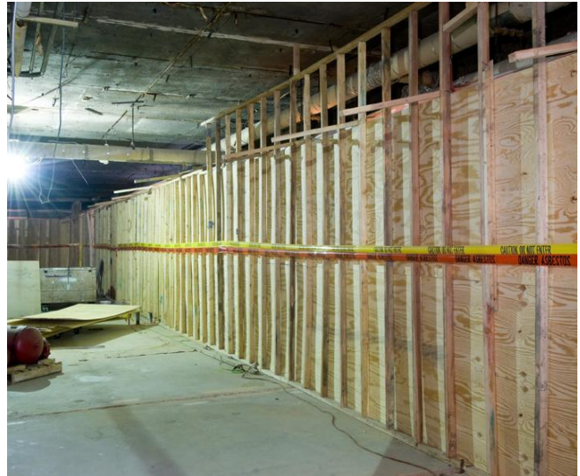
Figure 4: Existing 13 th Floor Abatement
