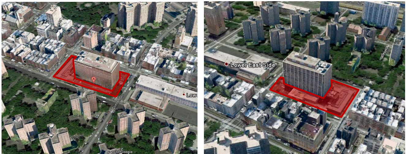
Figure 16: Front and Rear Existing Conditions View
